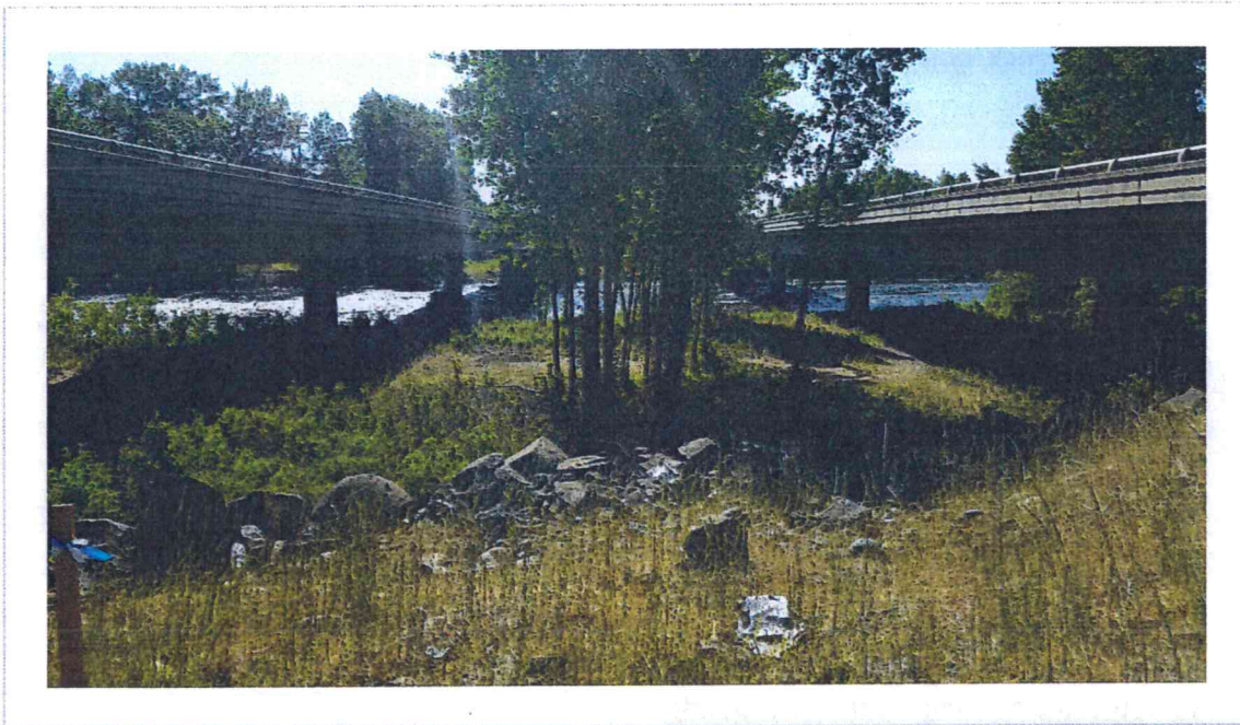
Photo 13 - Median looking east
